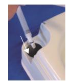
Due to the horseshoe shape of the flush tube, when refitted, the nozzle will be guided back up towards the hole at the entrance of the bowl.
