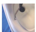
G. when pulling the nozzle through the hole, make sure that the small rib on the nozzle is pulled inside the toilet bowl.
